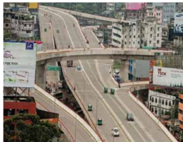
Financing in Mayor Md. Hanif Flyover Jatrabari, Dhaka
